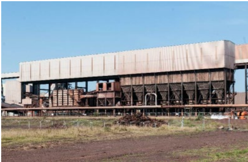
Plate 1: The stock house. Image taken from TEP, 2021, Teesworks Industrial Zone, Historic Building Recording
