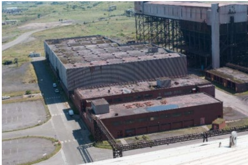
Plate 2: View of the area workshops with the stock house to the right of the view and the single-storey substation at the foot of the stock house
